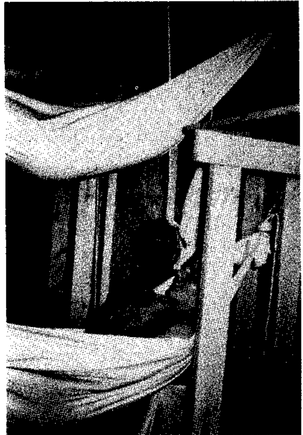
Fig. 14.4. Bedsheet-Hammocks hung one above the other across the room of a Russian-type Small-Pole Shelter made of lumber.
