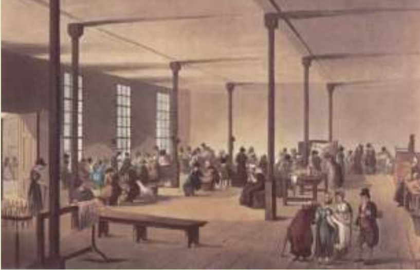
Workroom at St James Workhouse.
